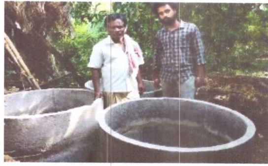
Installed Cement Ring
