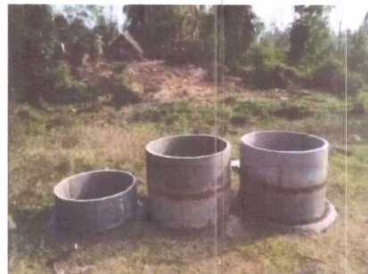
Installed Cement Ring
